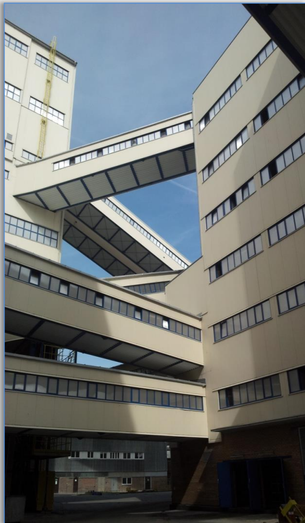
VIEW ON CONVEYOR BRIDGES CONNECTING FACILITY 101.1 WITH FACILITY 103.1/106.1
